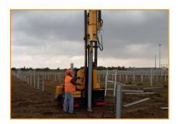
This foundation method requires analysis to understand the bearing capacity and corrosivity of the soil (performed by a Geotechnical Engineer). From an installation standpoint, specialized equipment and operators are required to install these types of foundations which increases the overall system costs.
