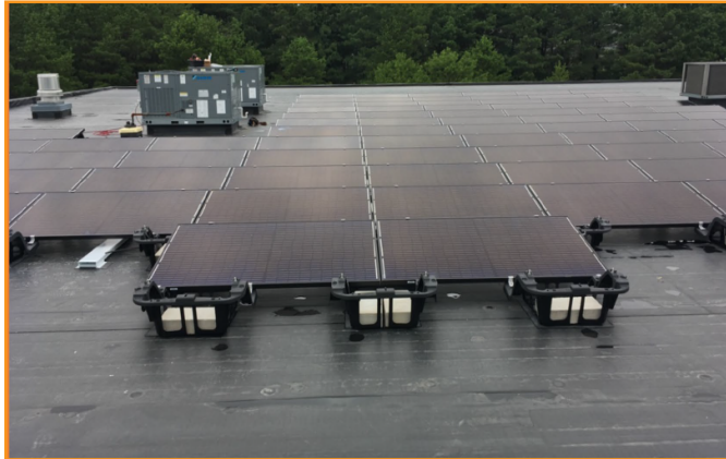
All wiring managed under module, BX chassis or in listed raceway.
