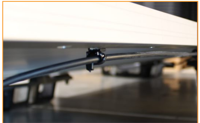
Examples of wire installation under module frame.
