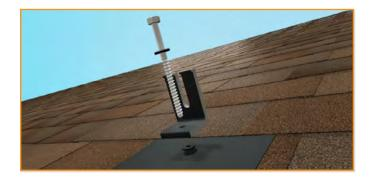
Drive lag bolt down into rafter using impact driver. Torque range is 100-400 in-lbs, depending on wood type and time of year. The EPDM on the bonded washer will push out the sides when compressed.
