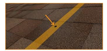
Slide flashing up under the next row of shingles directly above the pilot hole, taking care to align the hole in the flashing with the pilot hole.
