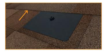
With the EPDM bonded washer threaded onto the lag bolt, followed by the L-Foot, insert the lag bolt into the gasketed hole in the flashing.
