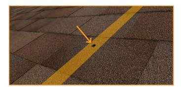
Slide flashing up under the next row of shingles directly above the pilot hole, taking care to align the hole in the flashing with the pilot hole.
