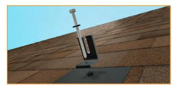
Drive lag bolt down into rafter using impact driver. Torque range is 100-400 in-lbs, depending on wood type and time of year. The EPDM on the bonded washer will push out the sides when compressed.
