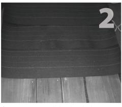
If necessary, remove shakes directly above mount with the roofing bar to expose felt paper. Flashing should reach at least 1 inch up and under the felt paper for proper waterproofing.
