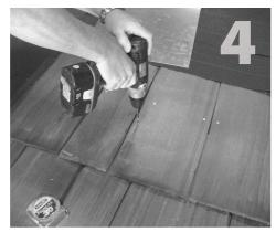
Set mount aside. Using drill with 7/32" bit, drill pilot hole into roof and center of rafter, taking care to drill square to the roof. Do not use mount as a drill guide.
