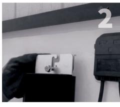
With the cap screw threaded into the bracket, slide the cap screw into the slot on the module level electronic mounting bracket with the bracket behind the module level electronic mounting bracket.
