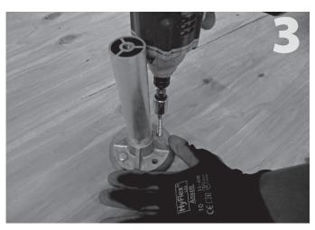
Prior to attaching the base to the roof, place the grade-8 hex bolt (item 1) in the bottom of the base (item 2) and screw the post (item 4) in. This is easier than adding the post after securing the base to the roof. Attach the base/post assembly to the roof with two lag bolts (item 3).
