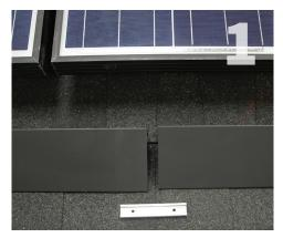
Lay out the skirt at the bottom of the array and complete any splicing if necessary. NOTE: clamps cannot be installed over the splice so be sure to account for this in layout planning.
