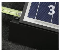
The QSkirt must extend a minimum of 1.2 inches past the edge of the module frame at the outermost corners of the array
