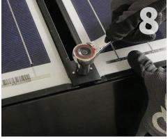
Using a 1/2 inch socket, tighten the clamp bolt onto the module. Tighten the clamp bolt to **12 ft-lbf**.
