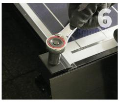
Using a 1/2 inch socket, tighten the clamp bolt onto the module. Tighten the clamp bolt to **8 ft-lbf**.
