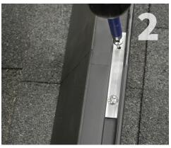
Slide the splice into the channel on the top of the QSkirt, and then slide an additional segment of QSkirt onto the splice. Press the two segments flush together and then slide the splice to line up with the screw holes. Fasten down the splice using the a #3 Phillips head screwdriver and the accompanying screws.
