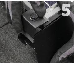
The End Clamp should be flush against the module frame. The lip of the upper clamp should be flush against the edge of module. Ensure that the lower section of the clamp body sits squarely on the top of skirt channel. The QSkirt should be flush with the front of the module.
