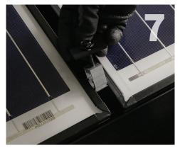
Connect the QSkirt to array using a Mid Clamp at each of the module breaks. Insert the Mid Clamp between the modules and rock it into position until it clicks into place. Take care that clamp head sits squarely on top of the module frame.
