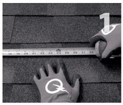
Locate, choose, and mark centers of rafters to be mounted. Measure vertical module dimension plus 3/4 inch to determine mount placement. Snap a line to aid with L-foot alignment.
