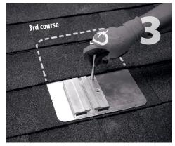
Insert flashing between 1st and 2nd course. Slide up so top edge of flashing is at least 3/4" higher than the butt-edge of the 3rd course and lower flashing edge is above the butt-edge of 1st course. Mark center of both holes for drilling.
