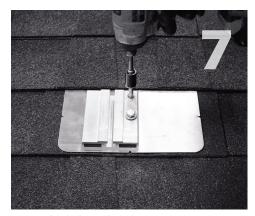
Prepare lag bolts with sealing washers. Using a 1/2inch socket on an impact gun, drive prepared lag bolts into the mounting holes. Driving the bolts in evenly is recommended. DO NOT over-torque or over-crush sealing washers.
