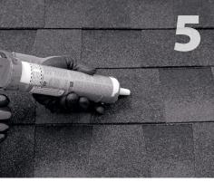
Clean off any sawdust, and fill hole with sealant Slide flashing into position. compatible with roofing materials.
