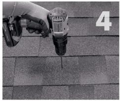
Drill pilot holes into roof and rafter using a with 7/32" bit, taking care to drill square to the roof. Do not use mount as a drill guide. Drill each hole 2.5" deep into rafter.
