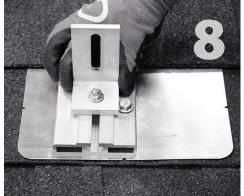
Using the racking kit hardware, secure the L-foot to the desired position on the mount. Torque racking HW to 13 ft-lbs.
