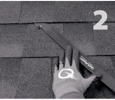
Carefully lift composition roof shingle with roofing bar, just above placement of mount. Remove nails as required and backfill holes with approved sealant. See "Proper Flashing Placement" on next page.
