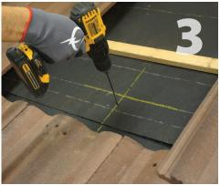
Drill two pilot holes using 1/8" bit to a depth of 23/4". Be sure lags go into center of rafter for strongest attachment. Pilot holes reduce rafter splitting. Fill pilot holes with appropriate sealant and align lag holes over the pilot holes.
