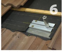
Use T-30 Torx bit and impact driver to secure mount Insert the grade-8 serrated flange bolt into the bottom of the post. Slide post into base plate channel. Line up post with the hole in the Universal Tile Flashing. Tighten post until snug with pliers.
