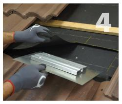
Waterproof at underlayment level according to roofing manufacturer instructions and Tile Roofing Association Guidelines.
