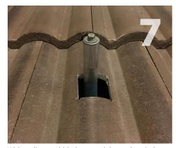
With a diamond blade on a right angle grinder or circular saw, cut tile to allow post to pass through. Place cut tile back in position. Insert post and tighten into place.
