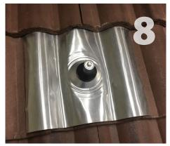
Install the 18"x 18" flashing. Pre-bend the flashing to follow the contour of the tile if curved. Apply sealant where post and flashing meet, and install EPDM counter flashing collar. Seal off the post from weather exposure with the racking hardware
